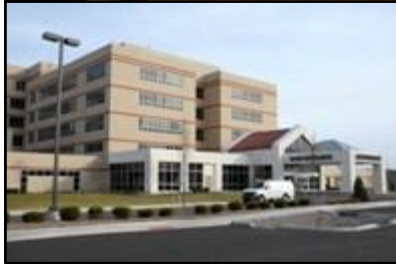
Top - Figure 3: Patient Rooms Bottom - Figure 4: Building Façade
